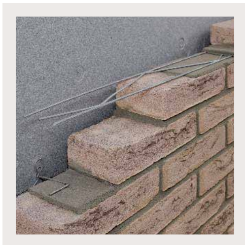
Armatura orizzontale WALL FORCE / Horizontal reinforcement WALL FORCE
